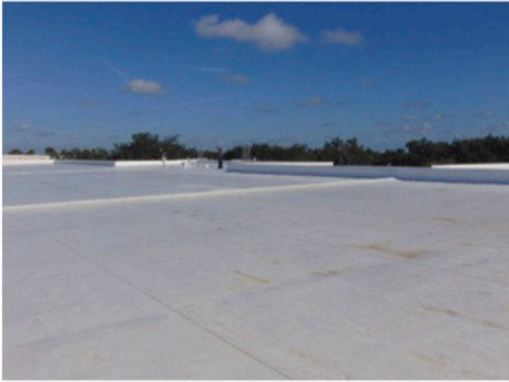
Reflective Roof Installation
