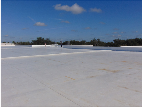
Reflective Roof Installation
